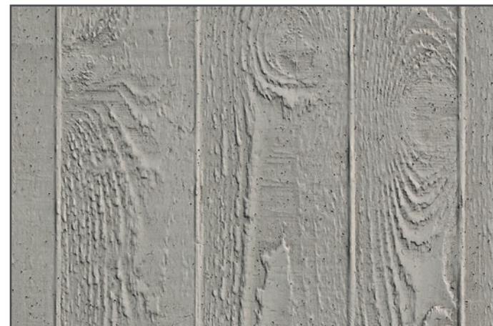
122 Brettschalung | timber formwork
